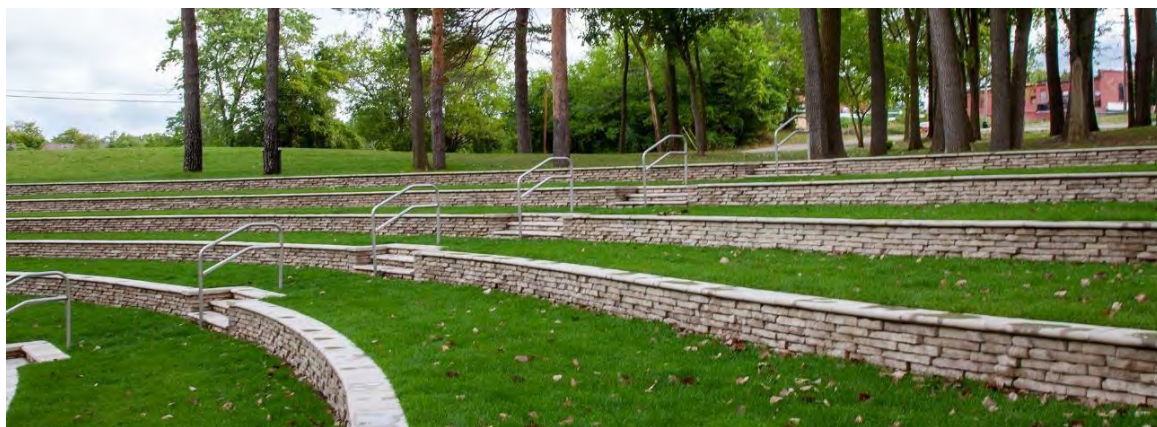
AMPHITHEATER VIEW (North West Corner)
